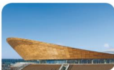
Velodrom Roofing membrane
