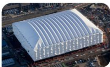
Basketball Arena Outer membrane
