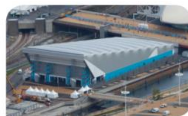
Water Polo Arena Outer & inner membrane
