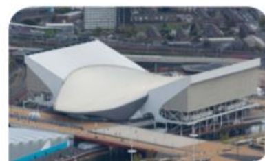
Aquatics Centre Outer membrane on "wings" & inner membrane
